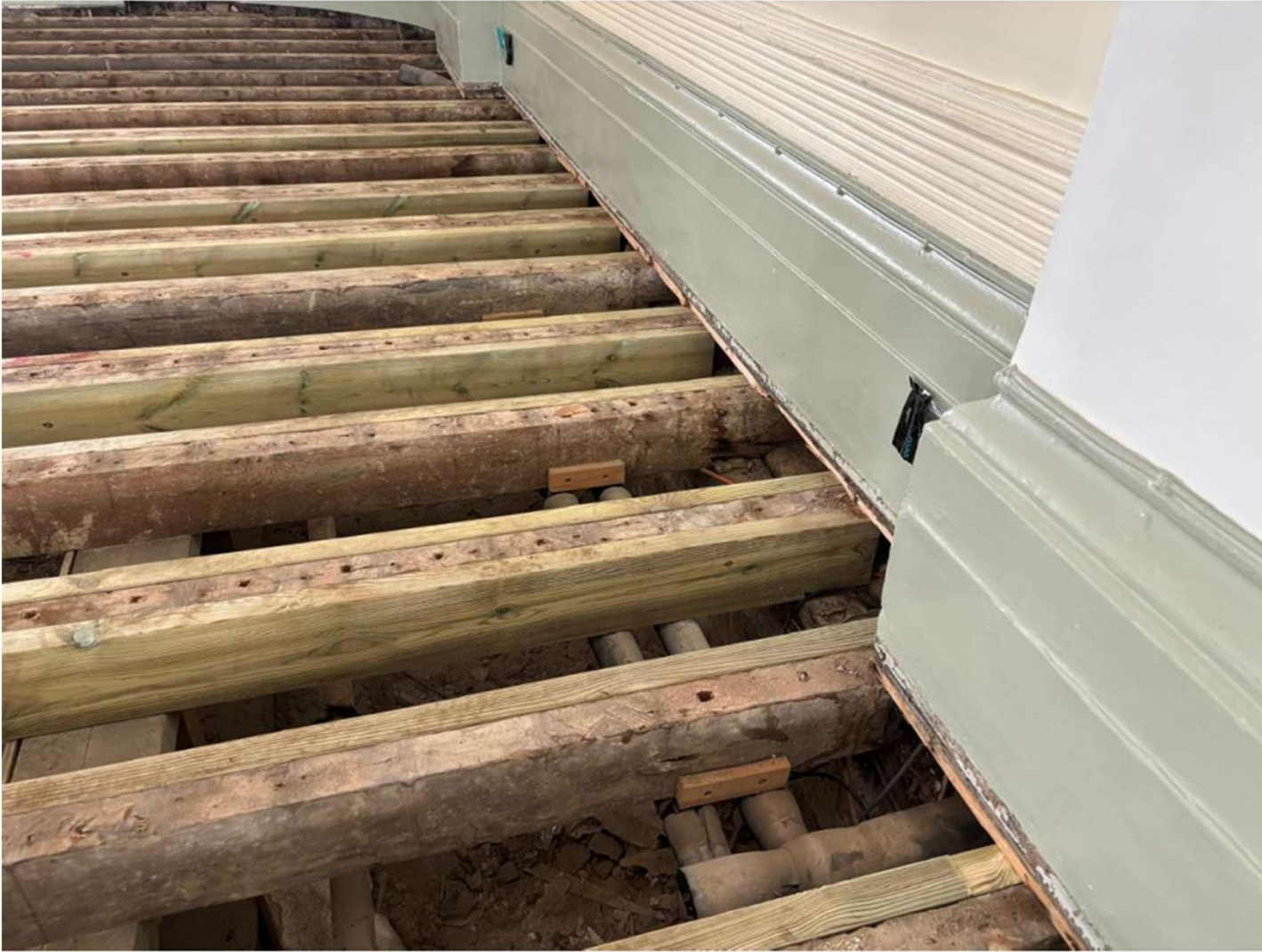
Figure 5. Close up showing the floor joists, where new joists have been fixed to the original joists.
