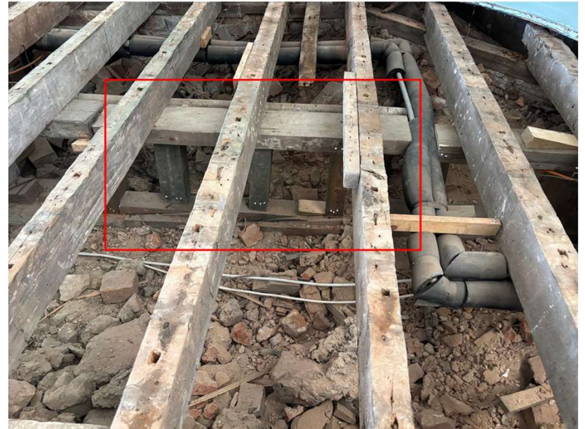
Figure 13. Works completed to headplate.
