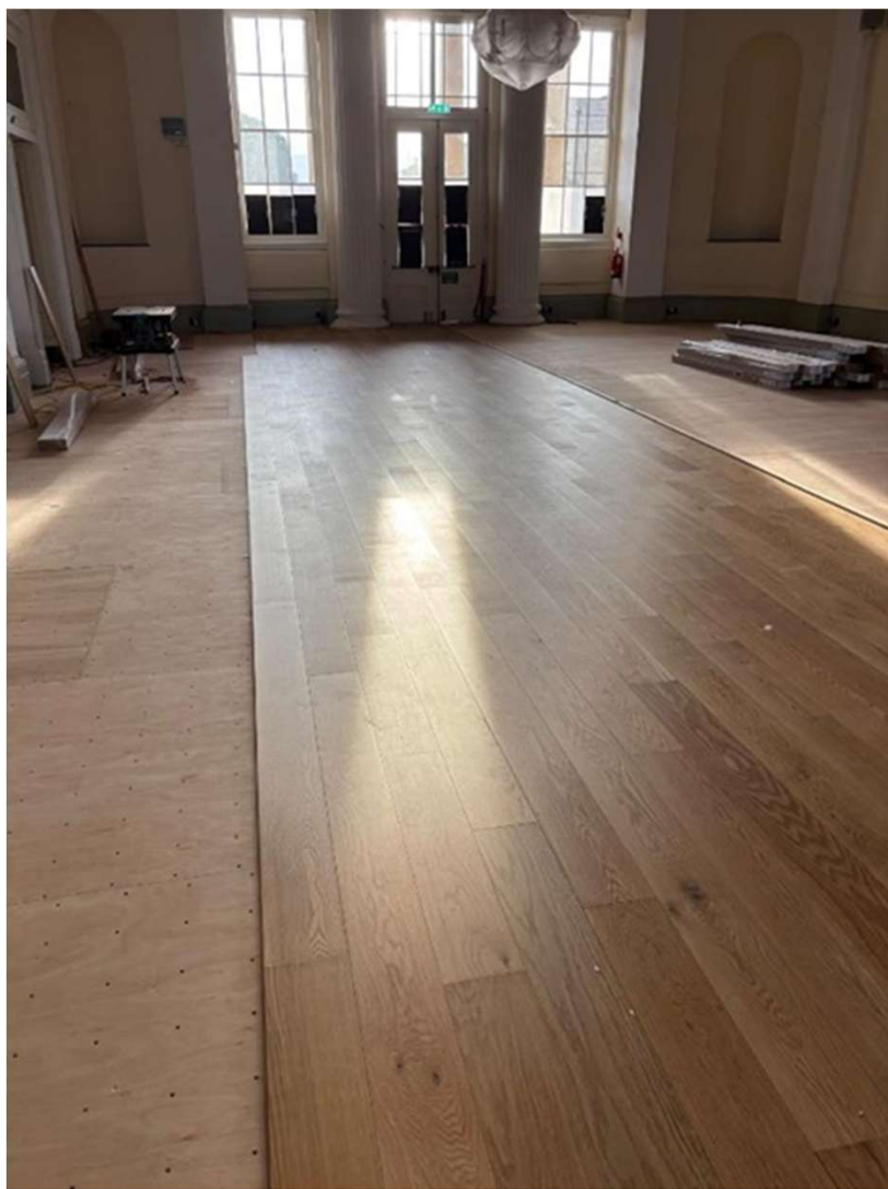
Figure 18. New floor deck in progress.
