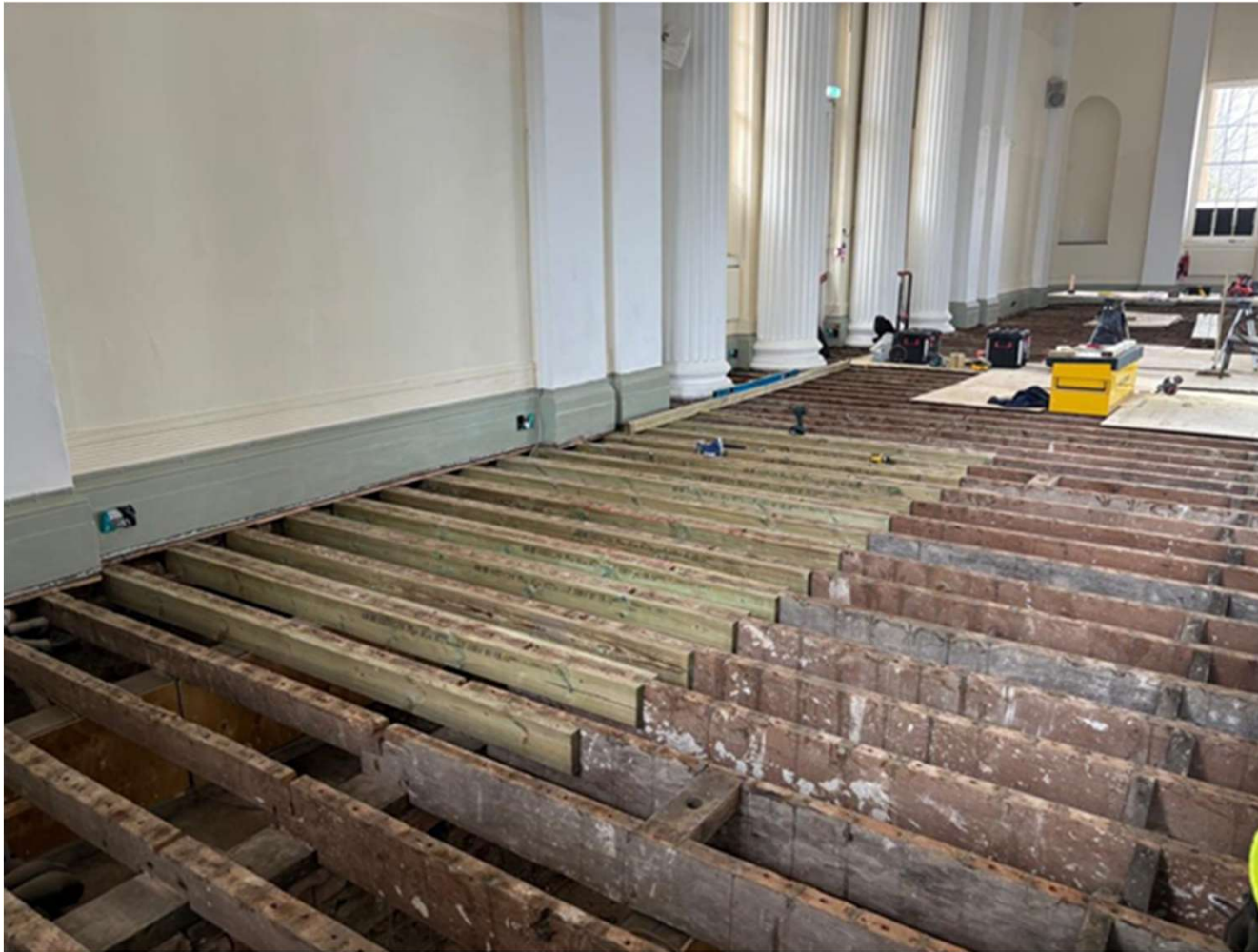
Figure 4. Floor strengthening works in progress. This photo illustrates where the original joists are being strengthened either with one additional joist or two. This method was continued throughout the main hall and apse as per the drawings.
