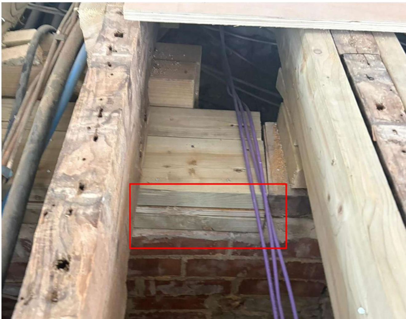
Figure 10. Timber replacement only where necessary. Timber affected by historic woodworm removed and replaced with new.
